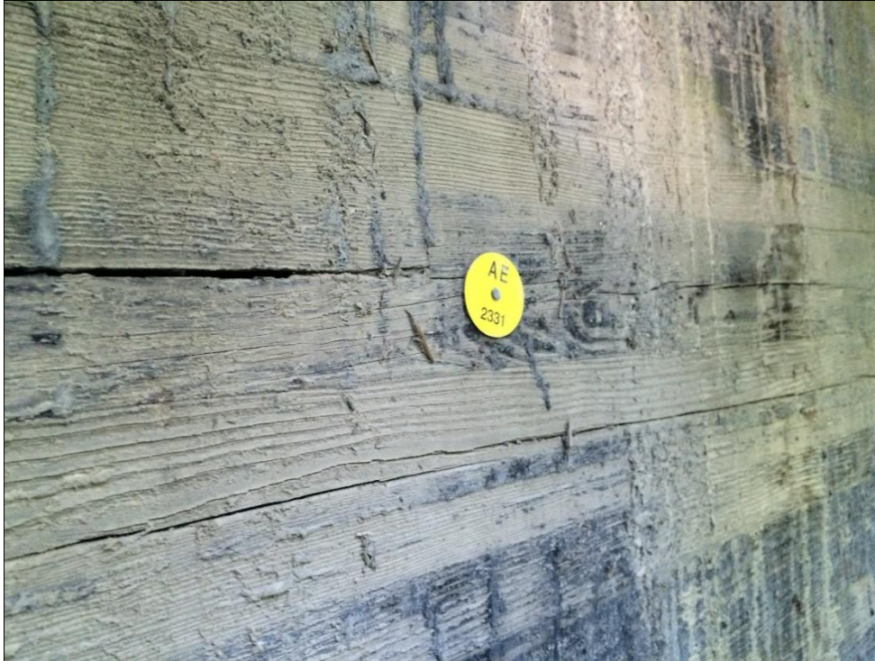
Photo #15 Girder 2, Exterior face
