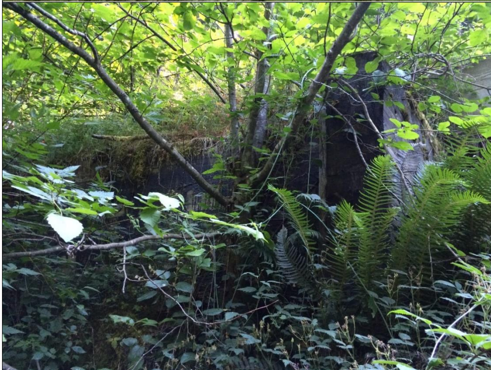
Photo #8 Camp End (A2), D.S. Wingwall / end of Ballast Wall
