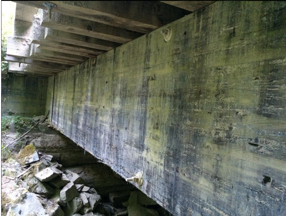
Photo #12 Girder 2, Exterior face
