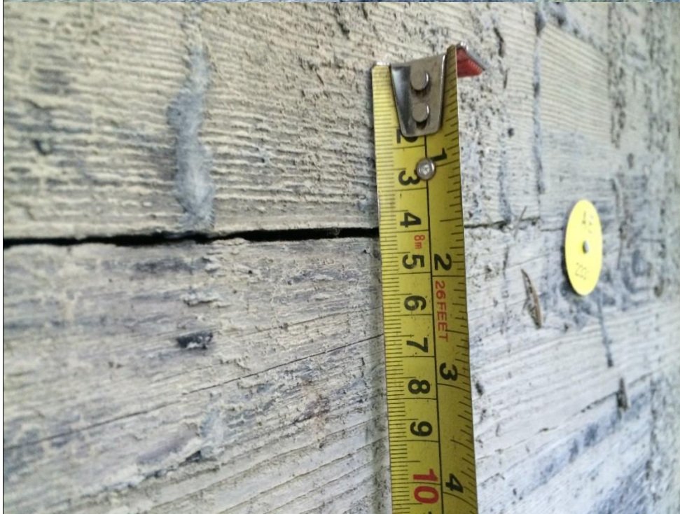
Photo #16 Girder 2, Exterior face
