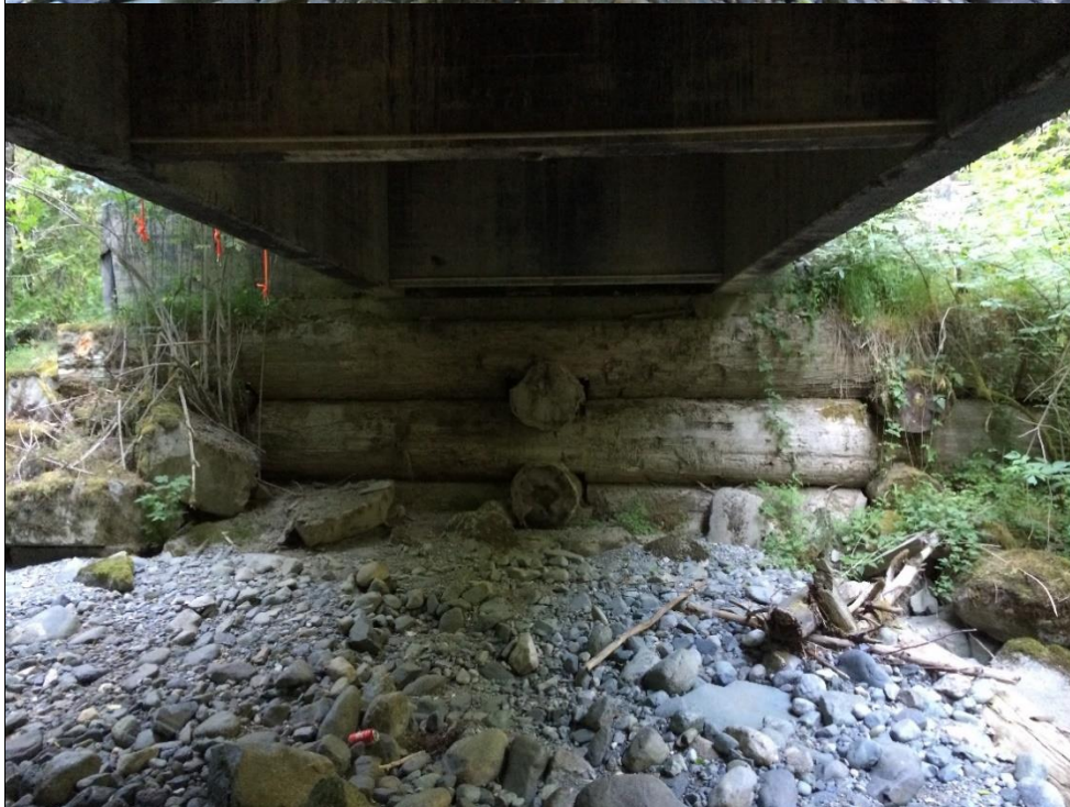
Photo #6 Woods End Abutment (A1)
