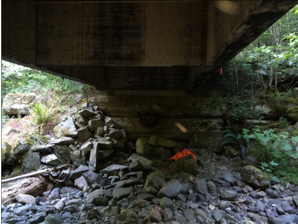
Photo #5 Camp End Abutment (A2)
