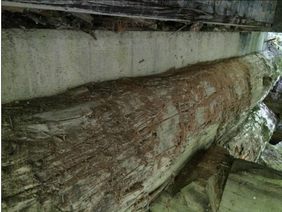
Photo #7 Camp End Abutment (A2)
