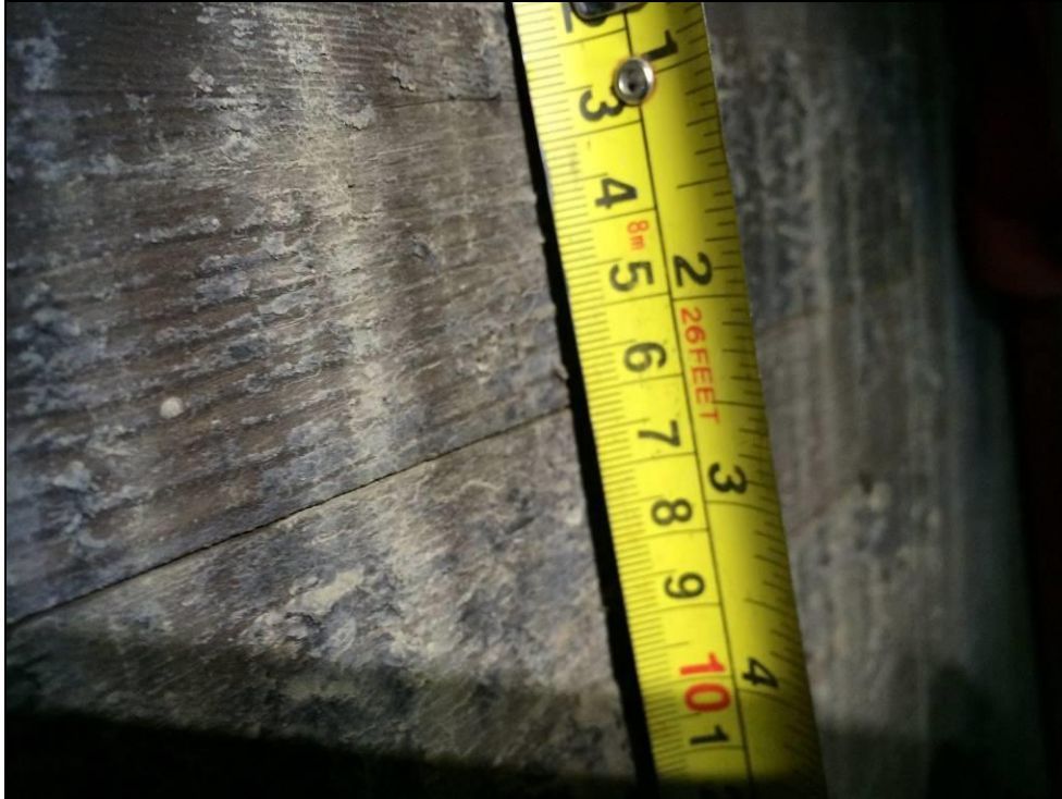
Photo #11 Girder 1, Interior face
