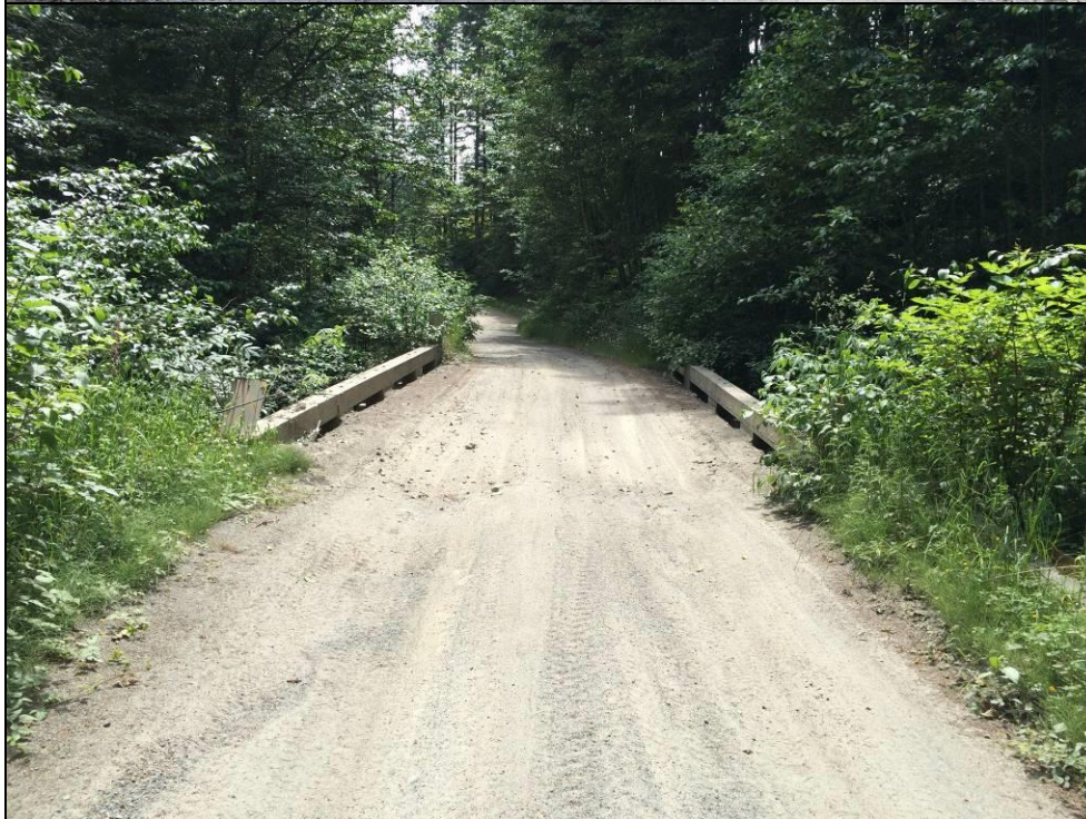
Photo #4 Woods End Approach
