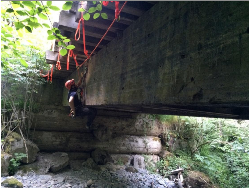
Photo #9 Girder 1, Exterior face
