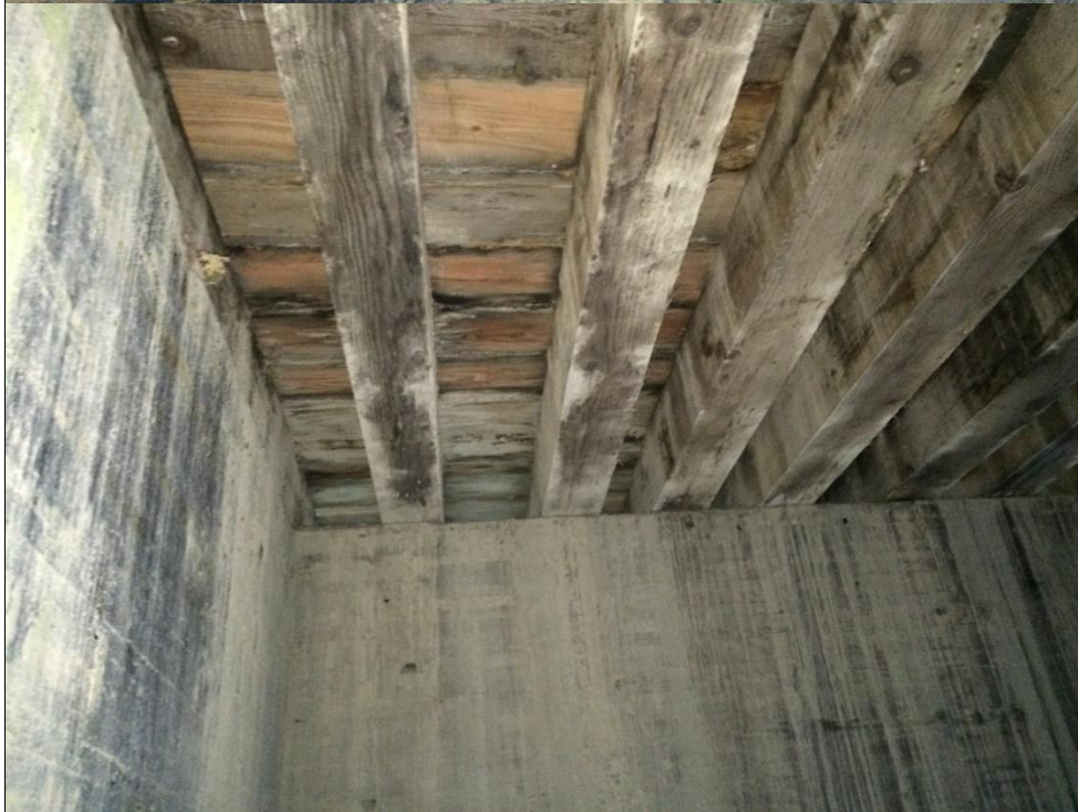
Photo #18 Typical underside of deck
