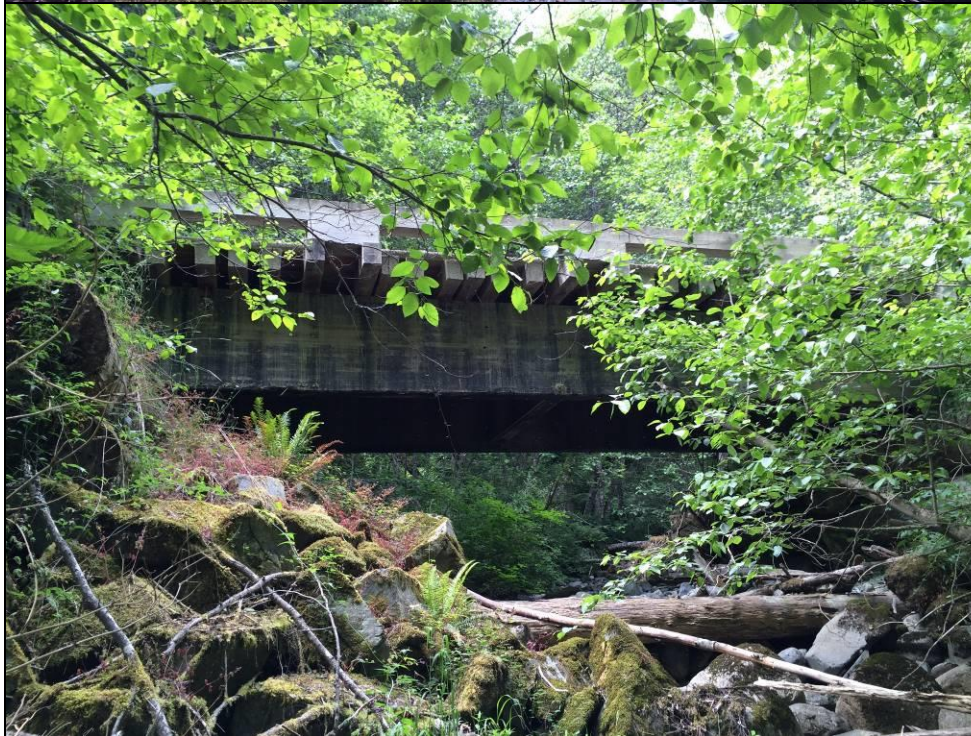
Photo #2 Downstream Elevation
