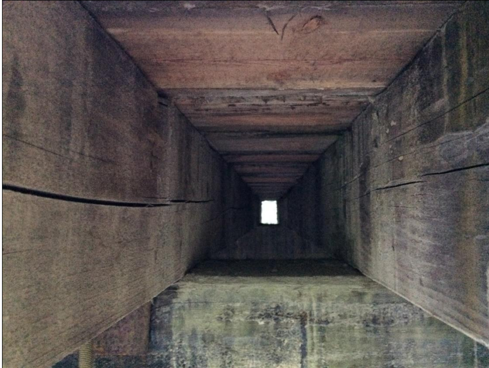
Photo #17 Typical space between transverse deck ties
